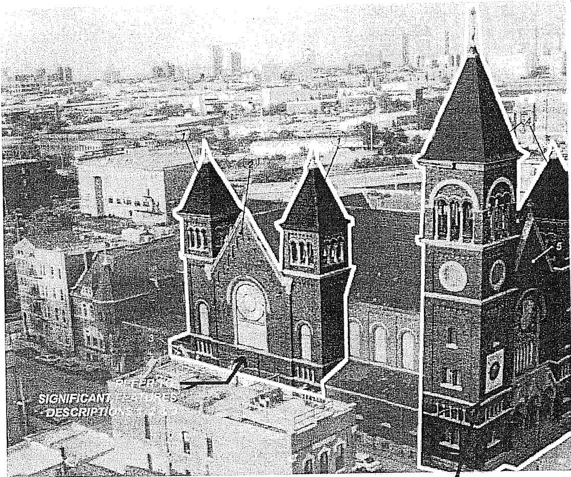
ST. BONIFACE CHURCH - WEST ELEVATION PORTIONS NOTED ARE SIGNIFICANT AND SHALL REMAIN, AND SHALL BE RESTORED
